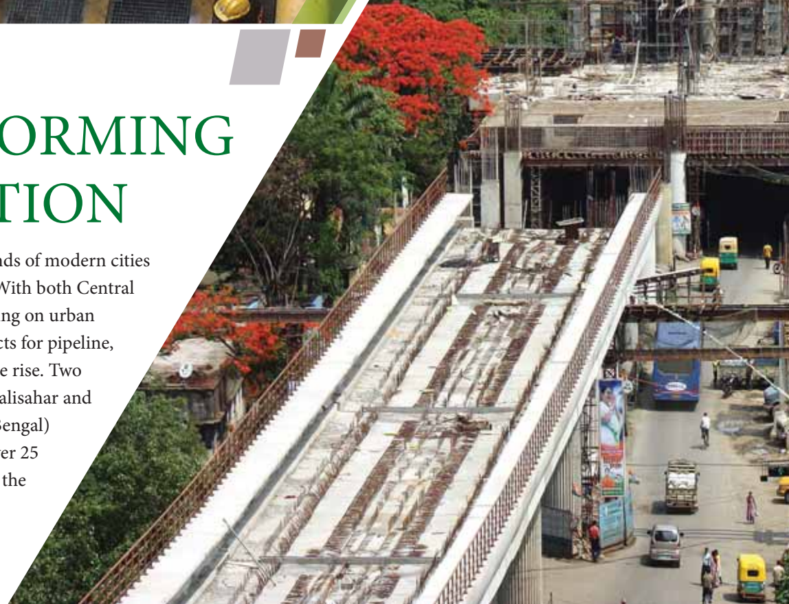
Aerial View of Joka Metro with one of Stations under Construction
