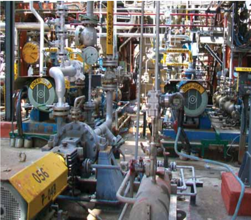
Pump, Exchanger, Vessel piping for IOCL, Digboi, Assam
