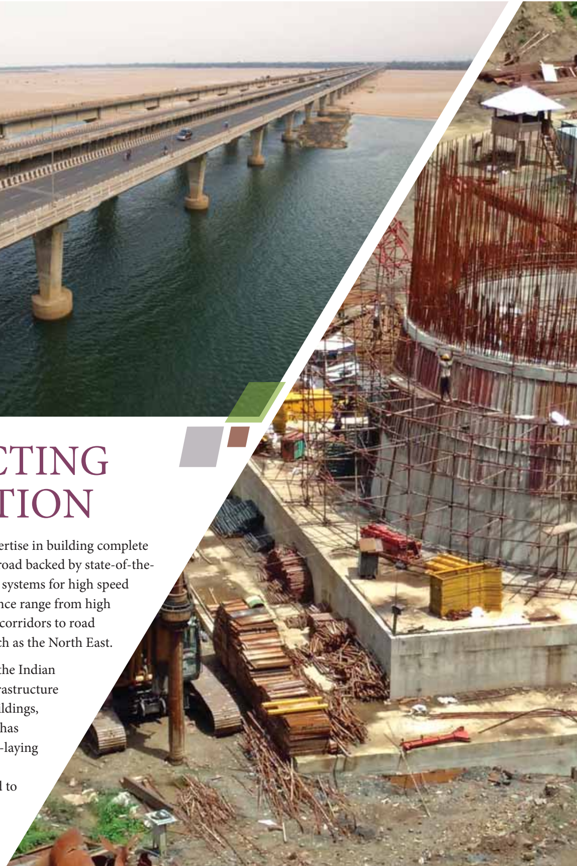
Under construction 141mtr high Railway Bridge at Manipur
