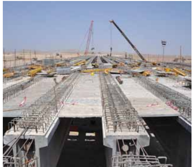
Bridge Construction in progress
