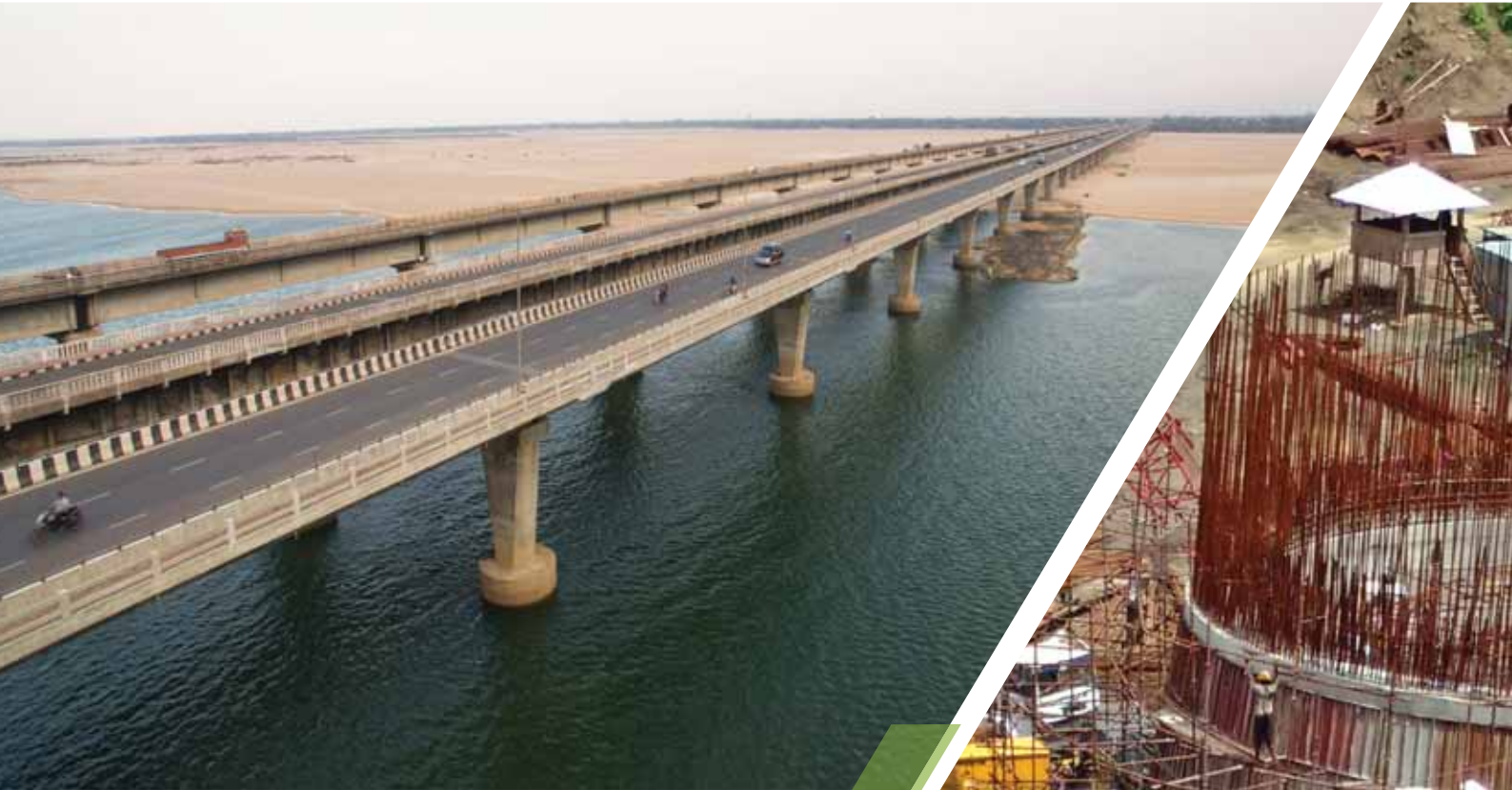
2.253 KM long Mahanadi River Bridge at Cuttack, Odisha
