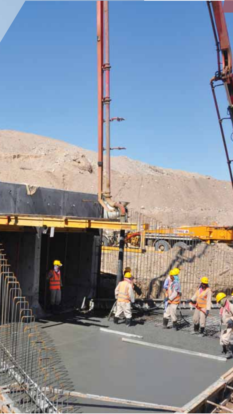
RCC Box Culvert work in progress
