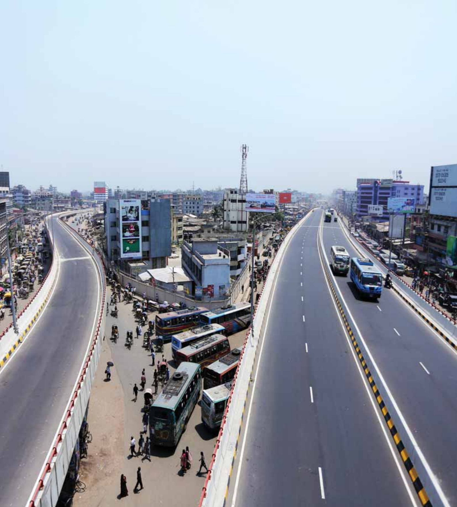
8 KM long 4 lane Jatrabari Gulistan Flyover at Dhaka, Bangladesh
