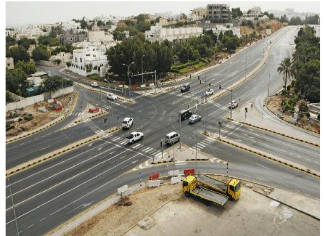
Ghubrah Bridge Widening Project at Muscat
