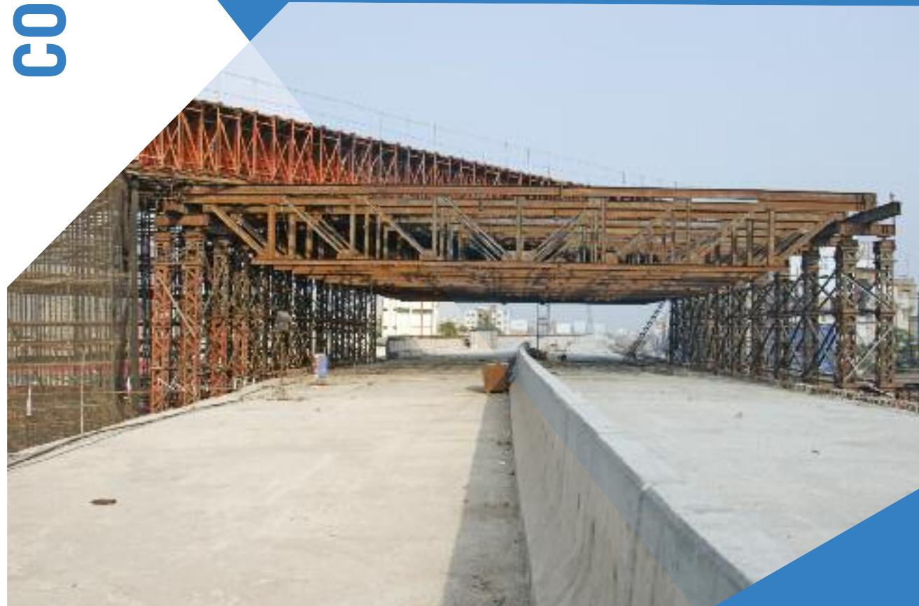
Another view of Jatrabari Gulistan Flyover in Bangladesh
