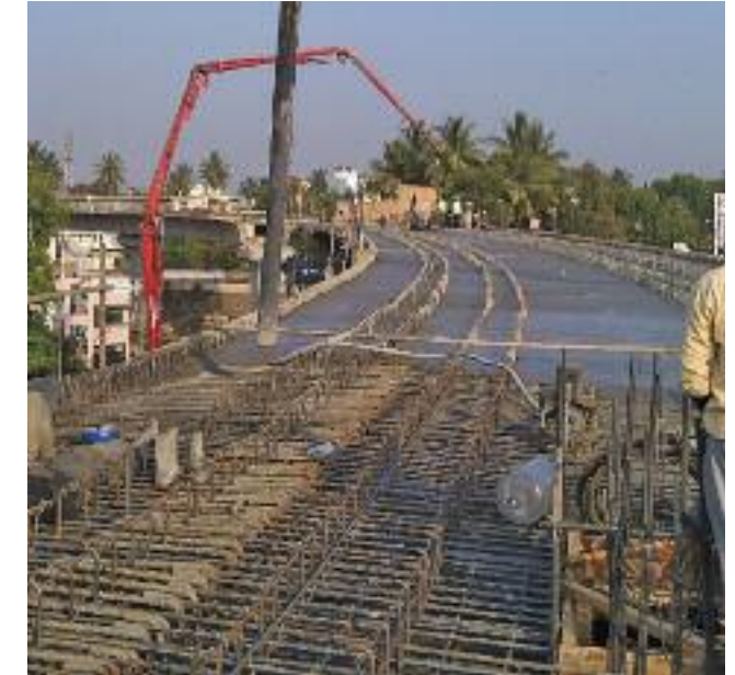
Construction of Bangalore Metro Project
