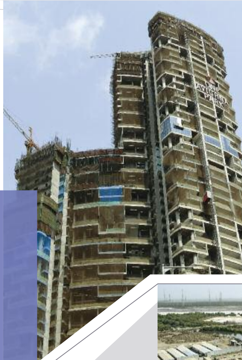
Civil Work for Residential Sale Towers including Podium at Avighna, Mumbai
