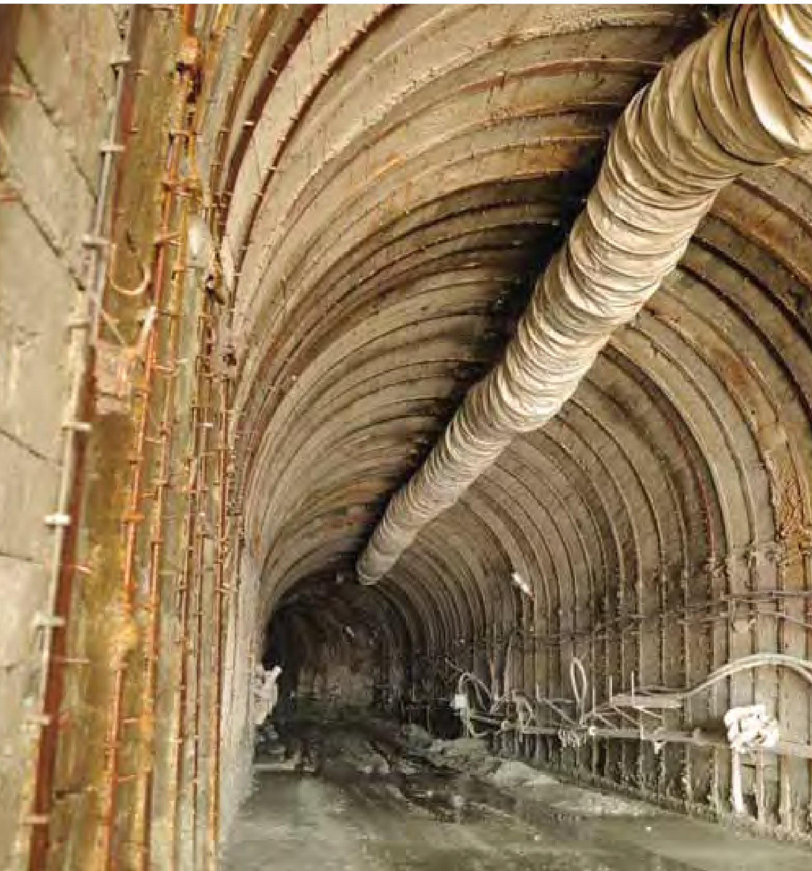
5.5 KM long tunnel construction for Bhasmey Hydroelectric Project, Sikkim
