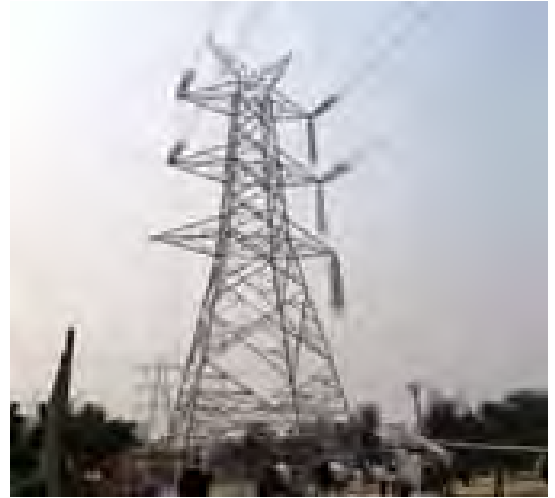
Construction of 400KV D/C QUAD Transmission Line from Siliguri to Bongaigaon
