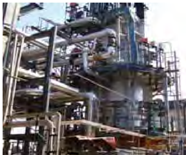
Piping and Equipment installation for MSQ Project IOCL Refinery, Digboi, Assam
