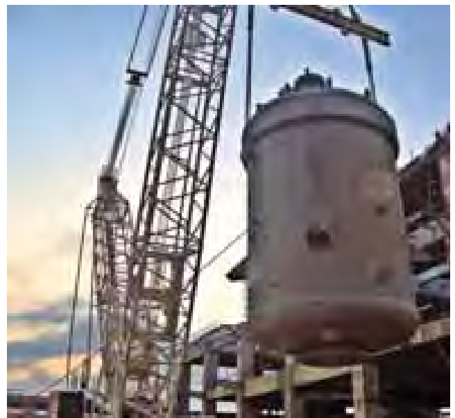
Erection of 90 MT Reactor for Polypropylene Unit of Phase III of OIL Refinery project for MRPL Mangalore, Karnataka
