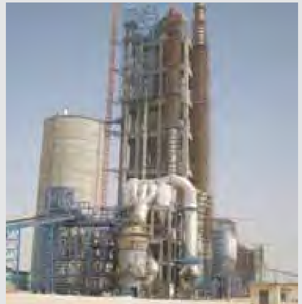
Cement Plant - UMM - BAB at Doha, Qatar
