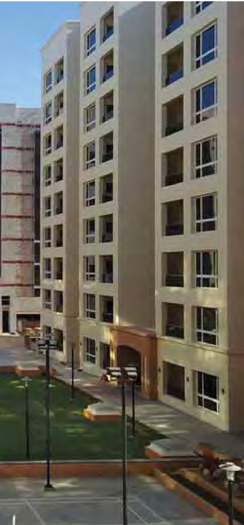
Construction of commercial / Residential Building (SAUD BHAVAN PLAZA) Muscat, Oman
