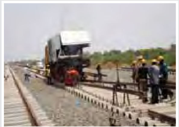
Imported flash – butt Welding Machine working for a track doubling project in A.P. for RVNL
