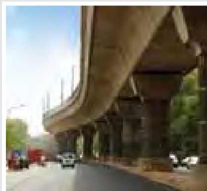
Metro Rail Project at Delhi
