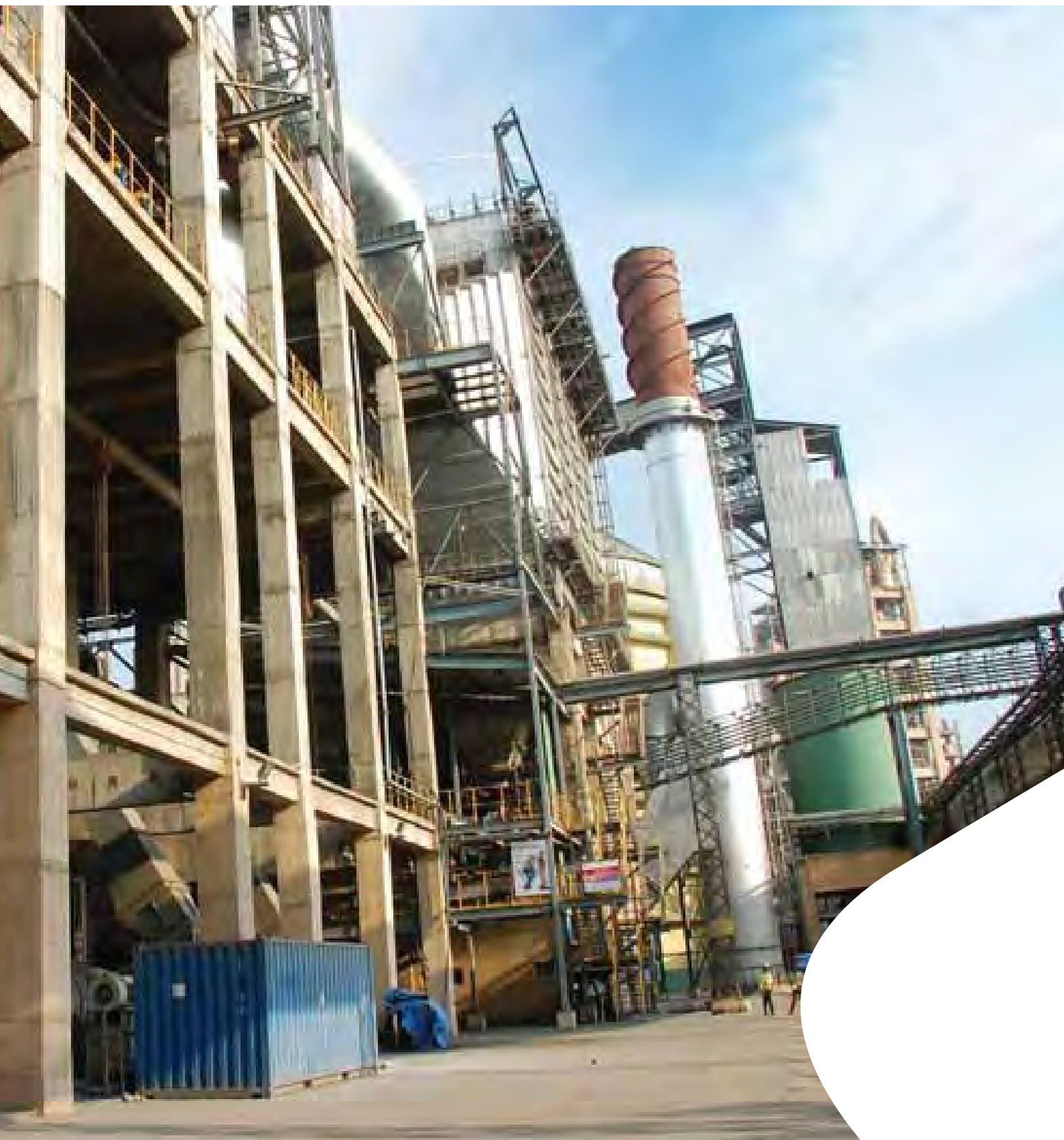
A view of Coal Mill Building for ACC Cement at Chandrapur, Chhattisgarh
