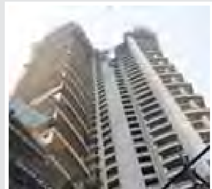
Construction of 64 Storied Residential Sale Tower at Mumbai
