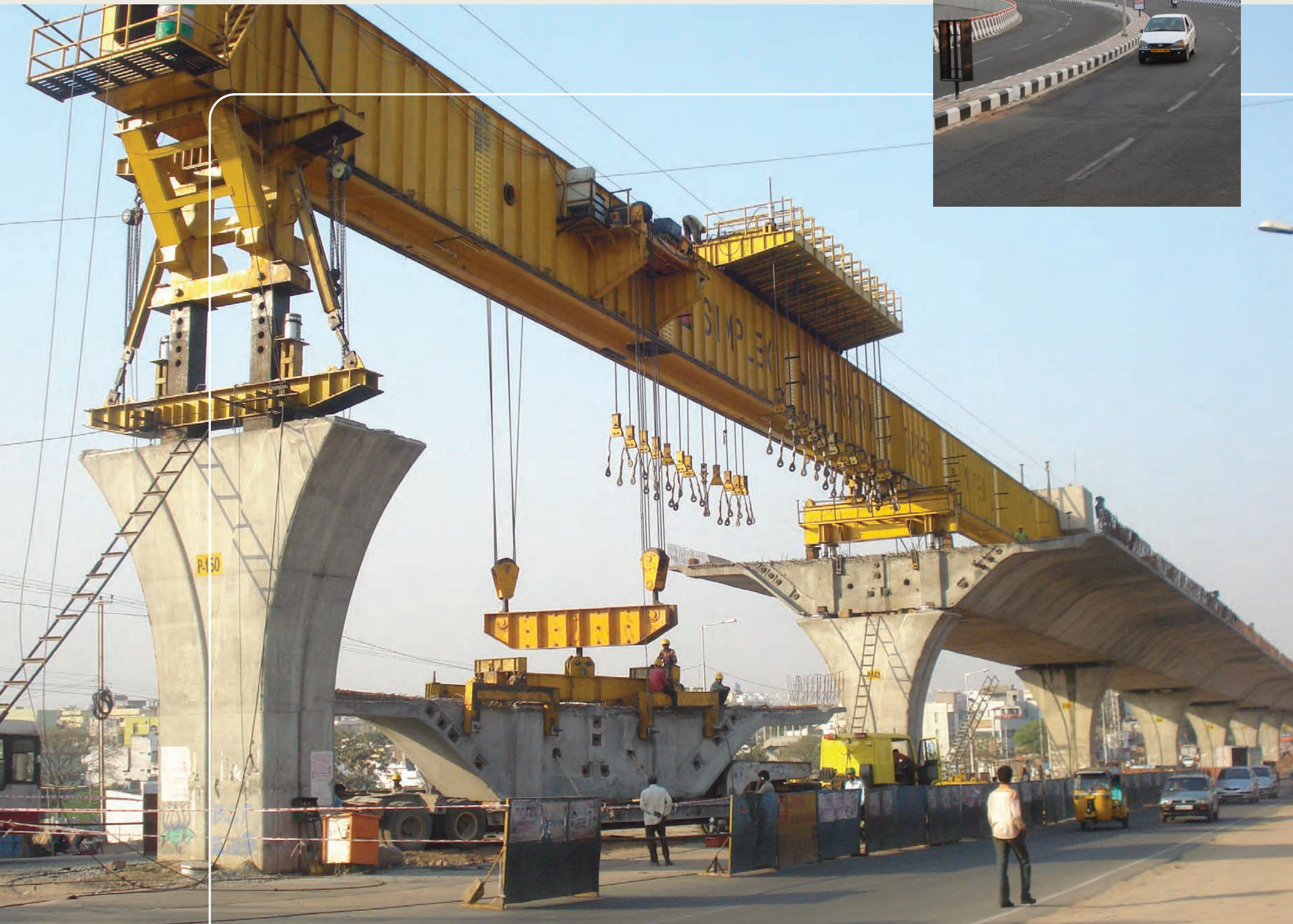
Pre-cast segmental construction of 17.2 Mtr. Wide, 11.5 KM long Narasimha Rao Setu at Hyderabad for HMDA
