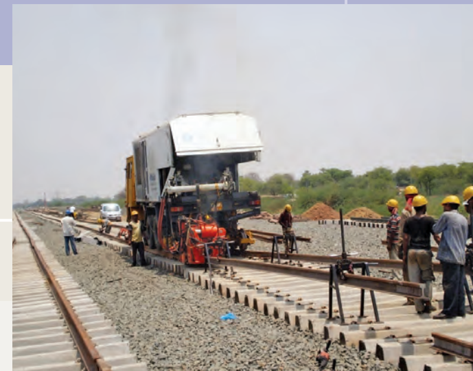
Fully automatic imported flush-butt welding machine working at Gooty-Pullampet track doubling project in Andhra Pradesh for RVNL.
