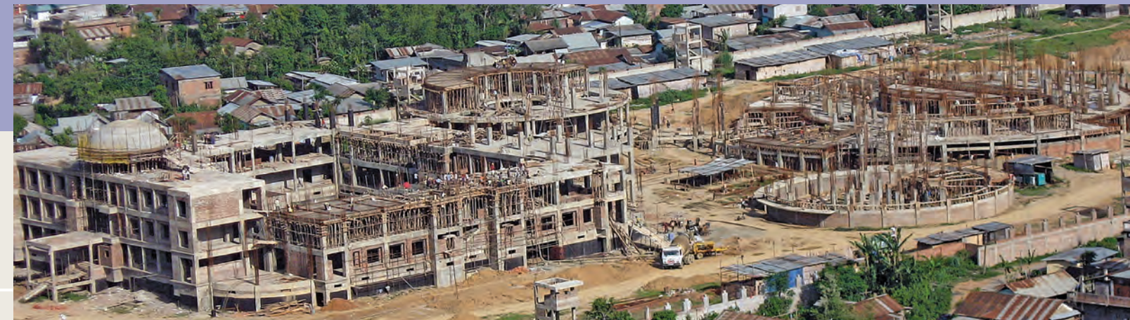
General view of construction of Assembly Complex at Imphal, Manipur – design and construction of civil, electro mechanical HVAC etc. by Simplex
