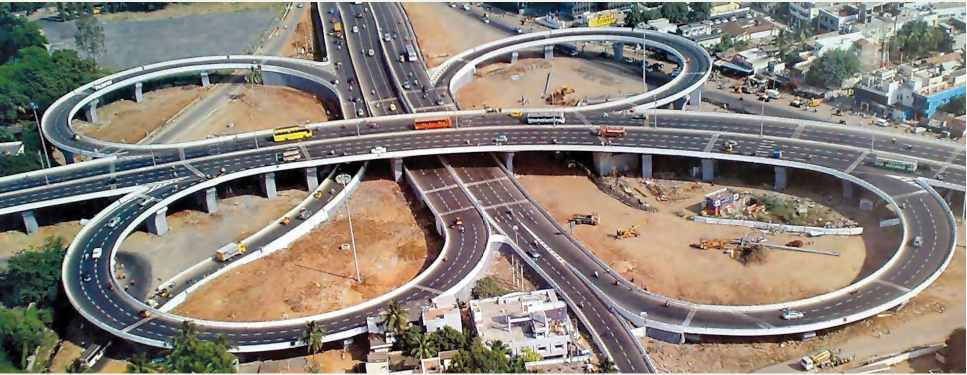
Flyover complex at Katipara Chennai for NHAI
