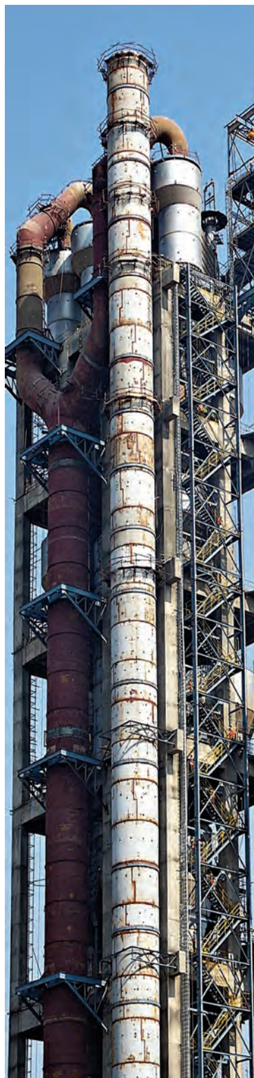
Pre-heater structure (110 m high) for a cement plant at Sonadih, Chattisgarh for M/s. Lafarge India Pvt. Ltd.
