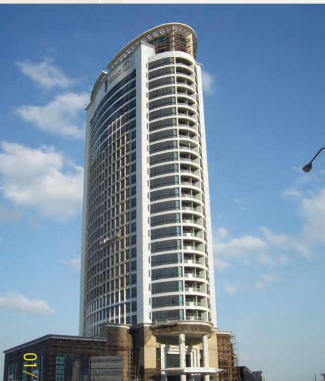
View of 26 storey Hilton Hotel at Doha, Qatar – complete civil construction by Simplex
