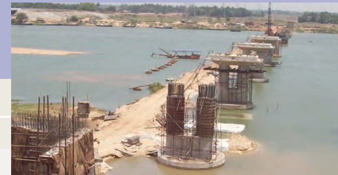
View of construction of bridge on river Mahanadi near Paradeep, Orissa for RVNL
