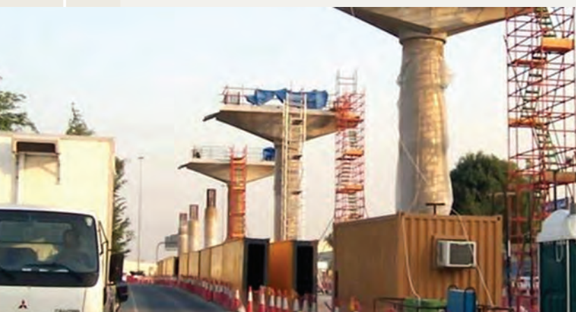
View of Metro Project under construction at Dubai
