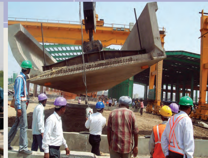
Manufacturing and Handling of precast pretensioned "U" girders for Mumbai Metro Project for M/s. MMOPL
