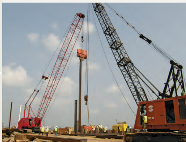
Piling operation at a major construction project site
