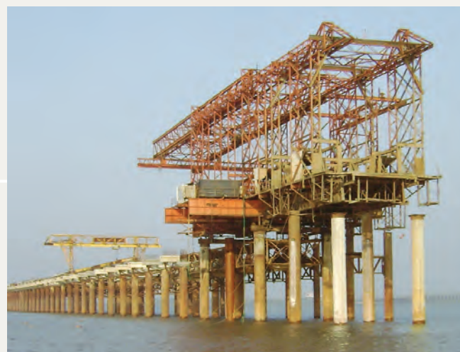
Construction of 1.2 km long approach bridge in sea in progress for Adani Petronet (Dahej) Port Pvt. Ltd., at Dahej, Gujarat
