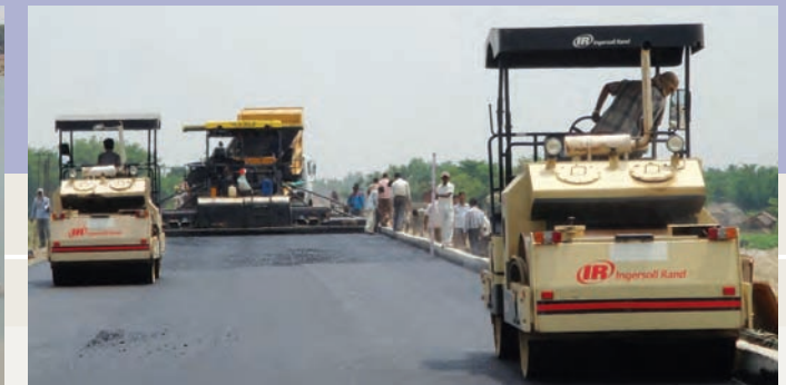
Road project under construction in Andhra Pradesh
