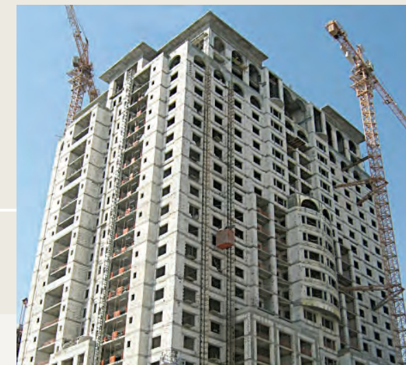
26 storied residential tower at Pearl Island, Doha, Qatar
