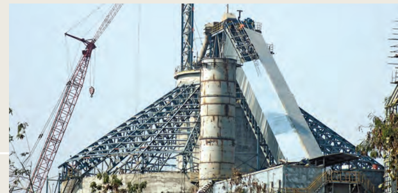
Erection of conical structural steel roof over clinker silo (45 m dia and 30 m high) for a cement plant at Sonadih, Chattisgarh for M/s. Lafarge India Pvt. Ltd.
