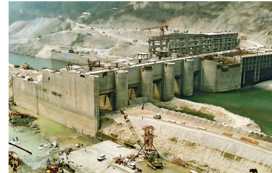
Teesta Low Dam Hydro-electric project under construction at Rambhi, West Bengal for M/s. NHPCL
