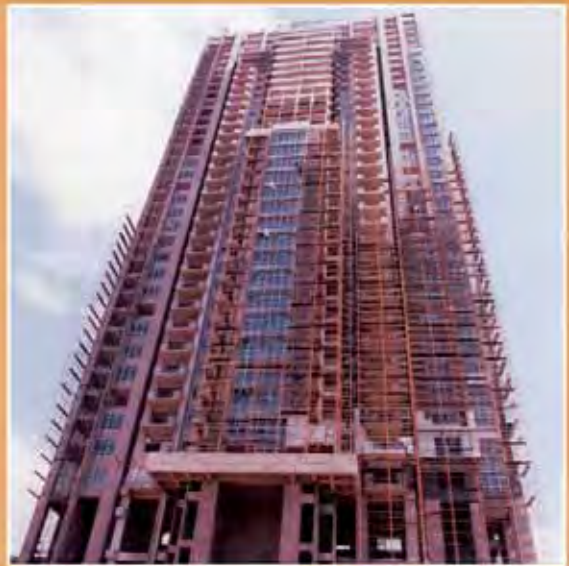
▲ Three residential towers of thirty five storeys each for M/s Sheth Developers Pvt. Limited at Pravadevi, Mumbai- Rs. 800 mn Imported MIVAN shuttering system was adopted resulting in extremely fast progress. As a result repeat order was received from the same client for several towers at Thane, Goregaon and Kandevelli- Rs. 1250 mn.
