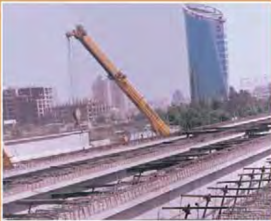
▲ Construction of flyover on NH-8 for NHAI in Delhi-Gurgaon section- Rs. 850 mn
