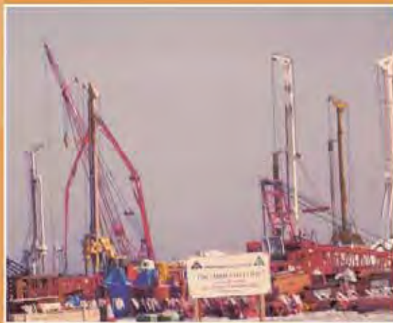
▲ 15 rotary drilling rigs installing about 10,000 bored piles round the clock for commercial cum residential complex at Doha, Qatar- Rs. 1430 mn
