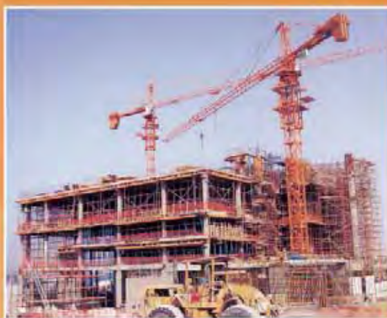
▲ Construction of twenty six storied Hotel Hilton at Doha, Qatar- Rs. 1074 mn
