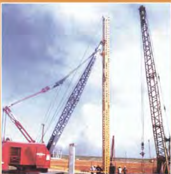
▲ Installation of 700 pre-cast jointed piles for construction of Providence stadium to host World Cup Cricket, 2007 at West Indies- Rs.120 mn
